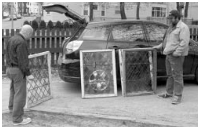
After restoration by Glenn Shalan, the Blake House leaded glass windows were ready for painting.
